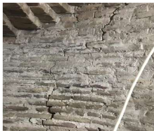
4-rasm. Binoning ichki devoridagi yoriqlar
